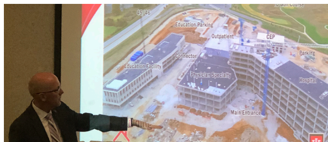
President of the IU Health South Central Region Brian Shockney with a panoramic view of the new Regional Academic Health Center under construction.
